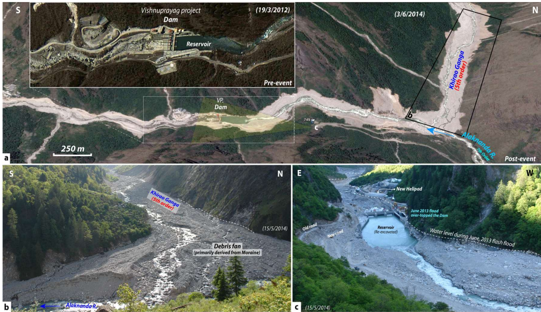
Fig. 1: (a) Pre- & post- June, 2013 event Google images showing debris flow along 5th order Khirao Ganga affecting Vishnuprayag project affected stretch of road and helipad ( inset ), (b) The debris fan and (c) the debris flow during flash floods overtopped dam and chocked the reservoir.
