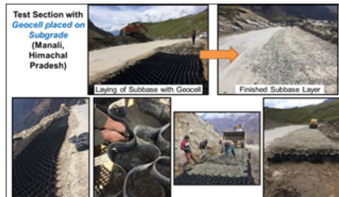
Laying of geocell reinforced pavement at NH-3, Manali-Sarchu road, Kullu District, Himachal
