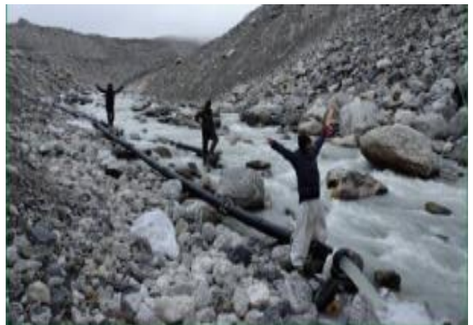
Source : SSDMA officials employing pipelines to siphon out water from South Lhonak lake (Source: http://www.ssdma.nic.in/Uploads/PdfFiles/glof.pdf ).
