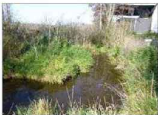
Water logging due to seepage
