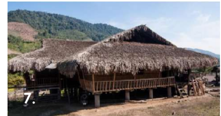
Bamboo & Cane House - Arunachal Pradesh; The example shows a Galo house, typically made of wood, bamboo, and cane, with roof made of toko leaves.
