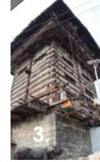
Koti-Banal - Uttarakhand; Alternating layers of stone and wood with high plinth and 3-5 storeyed structure
