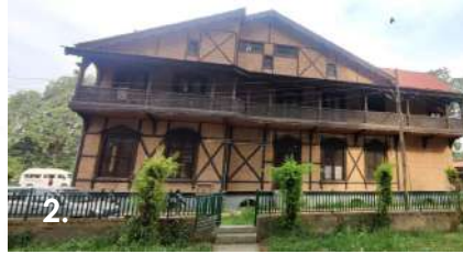
Dhajji-Dewari - Kashmir; Utilizes a timber frame filled with stone or brick masonry infill.
