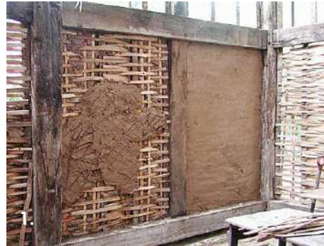
Wattle & Daub construction process
