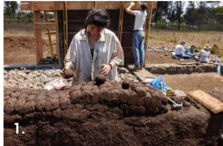
Mud Cob construction process
