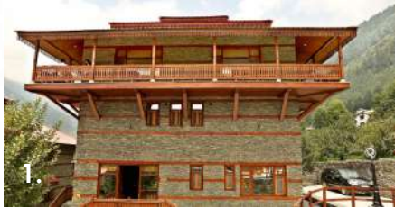
Kath-Kuni - Himachal Pradesh; Characterized by interlocking alternate layers of wood and stone masonry
