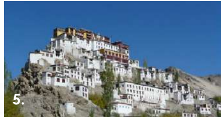
Adobe/Rammed Earth - Ladakh; Thick mud/adobe or rammed earth walls, flat roof and small windows with carved projected frames.
