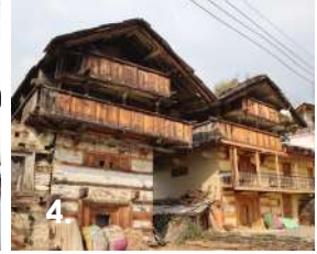
Koti-Banal - Uttarakhand; Alternating layers of stone and wood with high plinth and 3-5 storeyed structure
