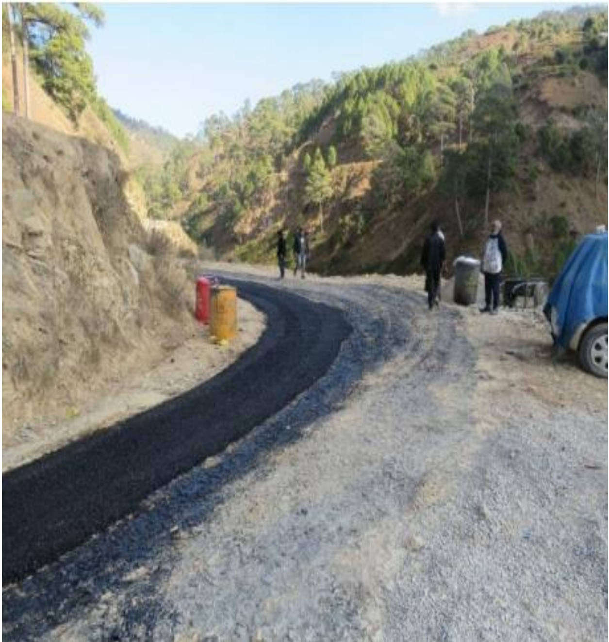
Laying of Bituminous Layer at Jhimar, Uttarakhand
