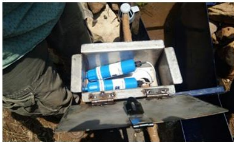
a) Water level sensors
