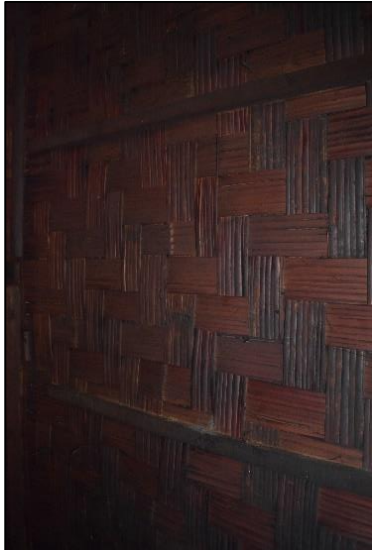
Fig. An: Ceiling
