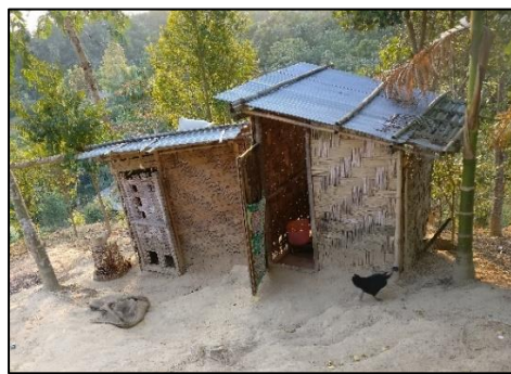
Fig. W: Bathroom made of bamboo
