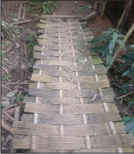
Fig. Y: Foot bridge
