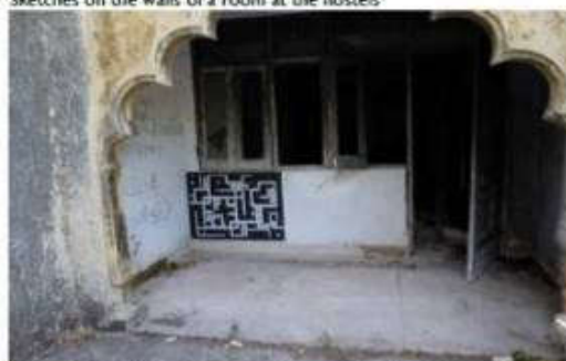
Entrance from the balcony to the rooms of the hostel
