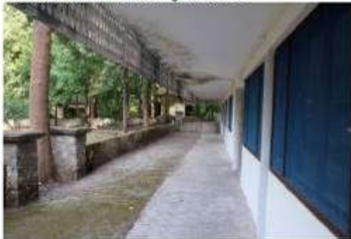
Administration building corridors
