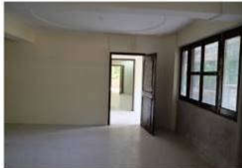
Inside the admin building
