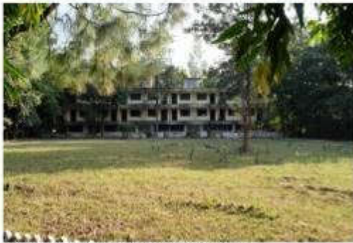
View of the administration building from outside
