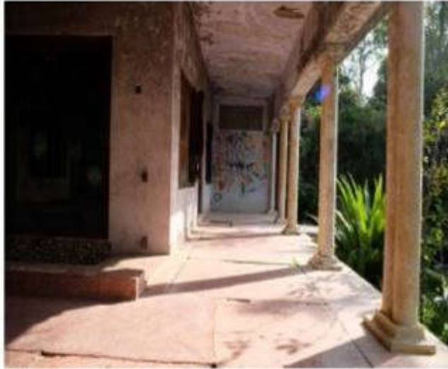
Art on the outer walls of the residence
