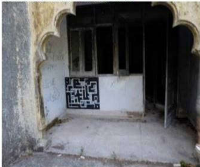
Entrance from the balcony to the rooms of the hostel
