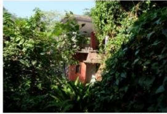
Building on site
