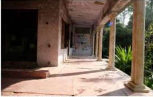
Art on the outer walls of the residence
