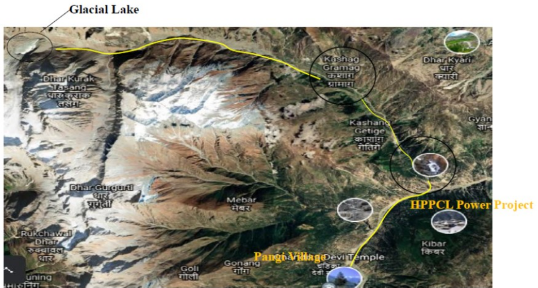
Figure 42. Vulnerable downstream locations in the Satluj river basin, Himachal Pradesh
