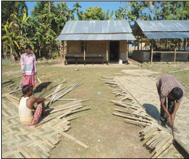
Removing the unwanted parts of the bamboo wall
