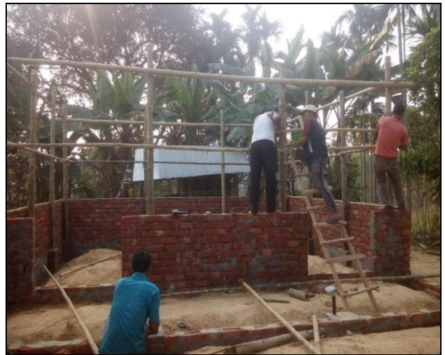
The house with the internal bamboo structure
