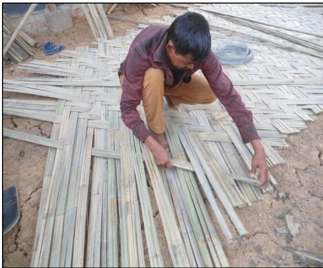
“Champa bain”: The traditional process of bamboo wall construction
