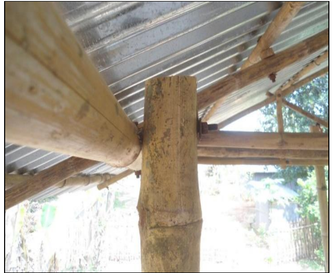
A section of bamboo can be used in case a bolt length go excess
