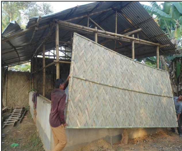
Fitting of bamboo wall on the house
