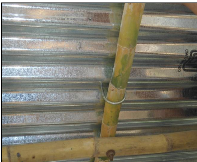
3: Putting metal cap, bitumen washer on the J-Hook and fastening it with nut
