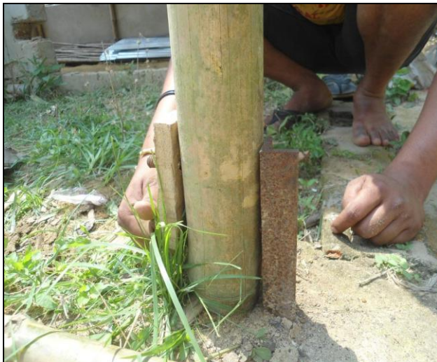
3: Fixing the pole with the iron angle
