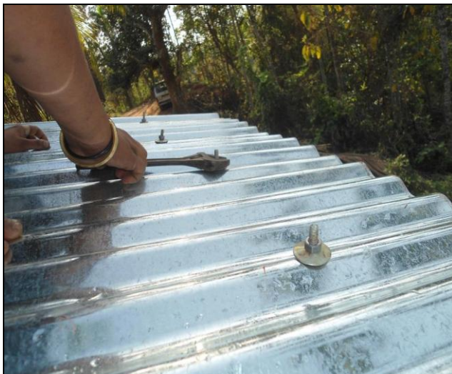
3: Putting metal cap, bitumen washer on the J-Hook and fastening it with nut
