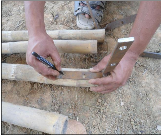
1: Marking on the bamboo
