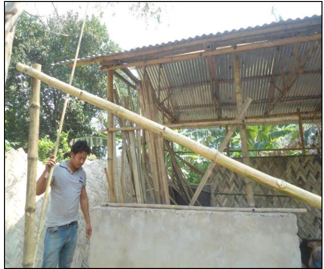
6: Fixing the horizontal bar/purlin at the veranda
