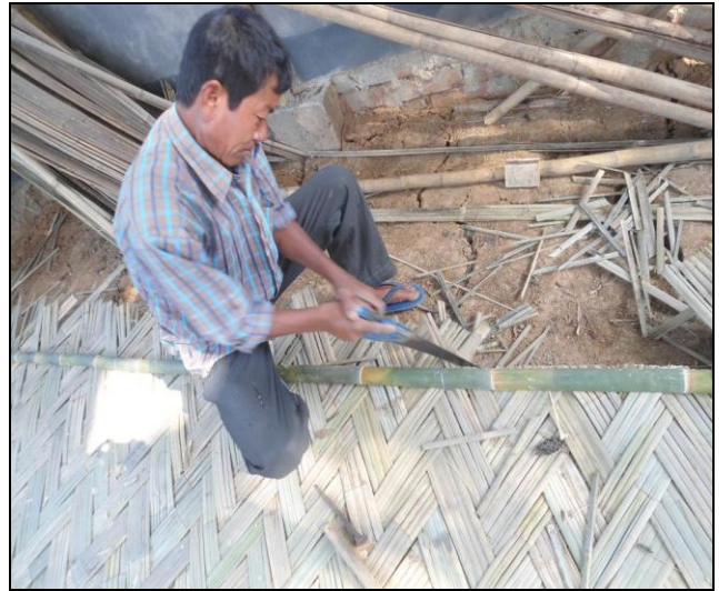
Removing the unwanted parts of the bamboo wall
