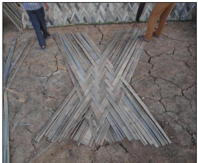
Making the frame on which the bamboo wall to be made
