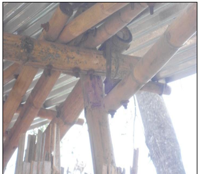
Joining of truss with horizontal bars
