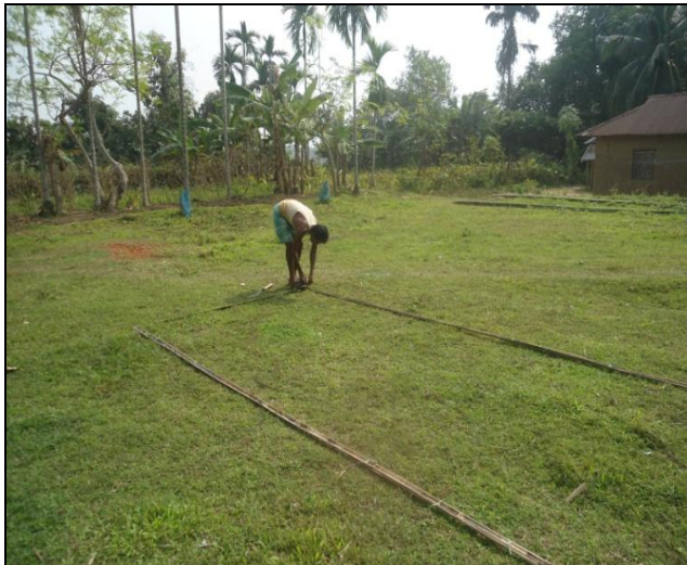
Making the frame on which the bamboo wall to be made
