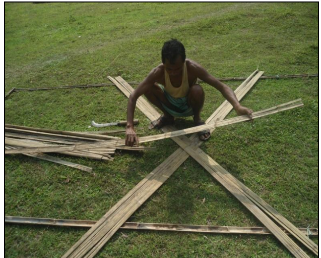
Making the frame on which the bamboo wall to be made
