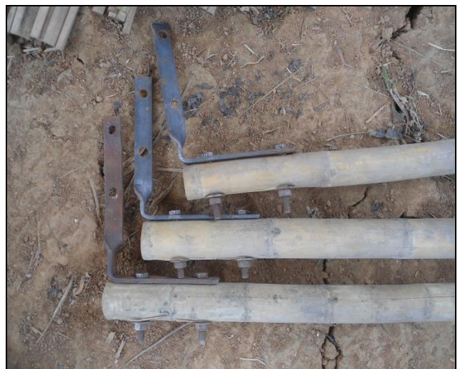
5: Kanakaich bamboo fixed with the clamp
