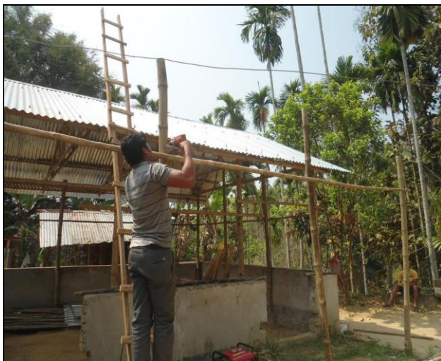
5: Fixing of the horizontal bar/beam/purlin
