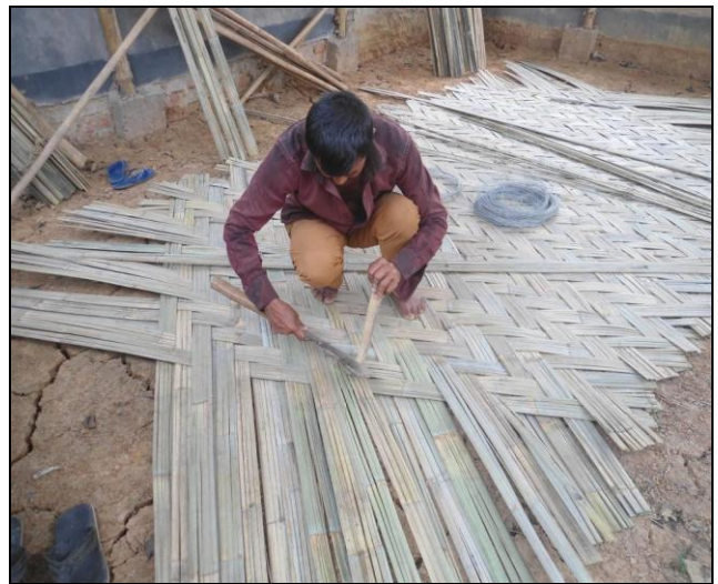
“Champa bain”: The traditional process of bamboo wall construction
