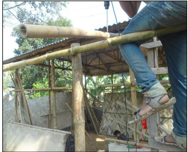
7: Joining of the clamp fixed on Kanakaich bar with the truss on the main building
