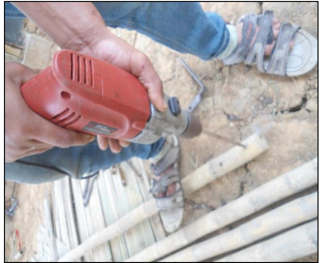
2: Making holes on the bamboo
