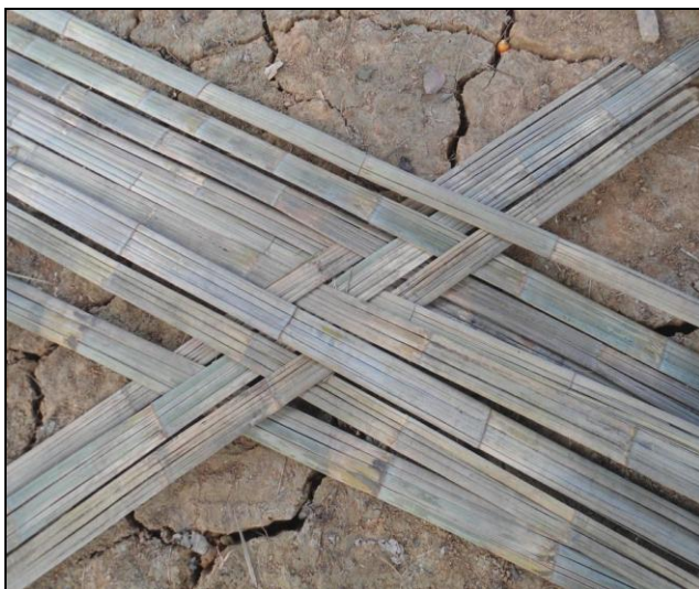
Making the frame on which the bamboo wall to be made
