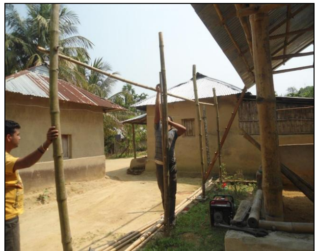
5: Fixing of the horizontal bar/beam/purlin
