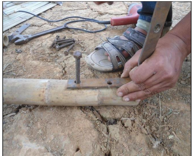
3: Placing the L-shaped clamp and insertion of bolt
