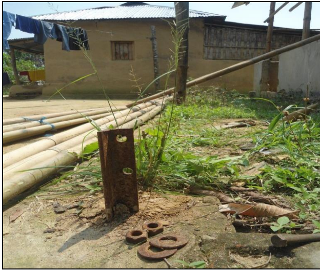
1: Fixed iron angle with the foundation
