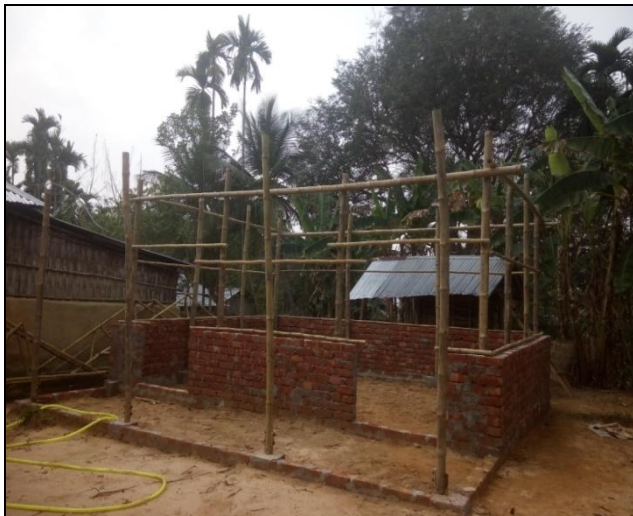
The house with the internal bamboo structure
