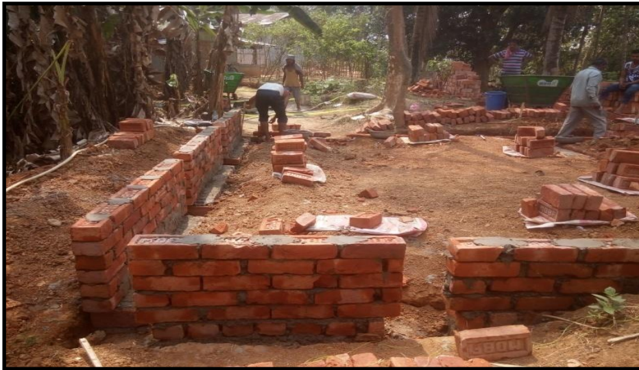
Raising of the bricked wall
