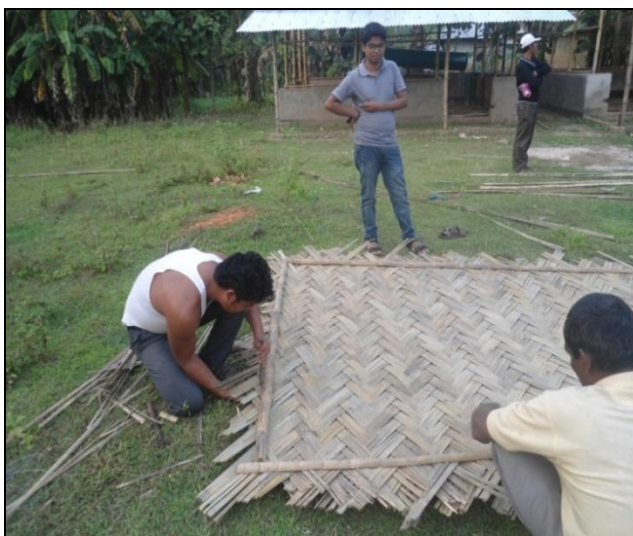
Tightening the wall structure by GI wire
