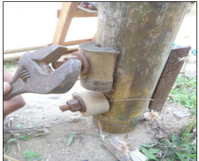
4: Tightening and aligning the pole
