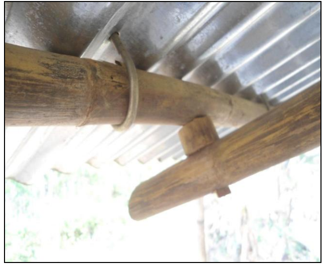
A section of bamboo can be used in case a bolt length go excess
