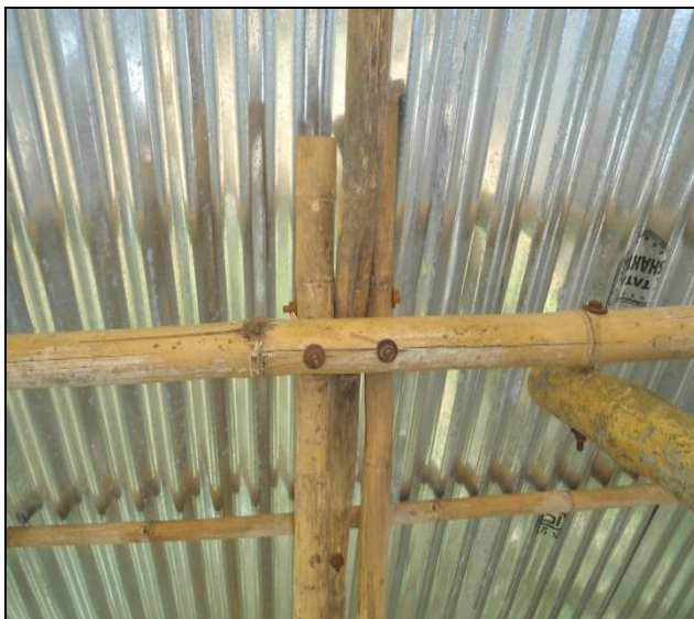
Joining of truss with horizontal bars
