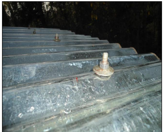
3: Putting metal cap, bitumen washer on the J-Hook and fastening it with nut
