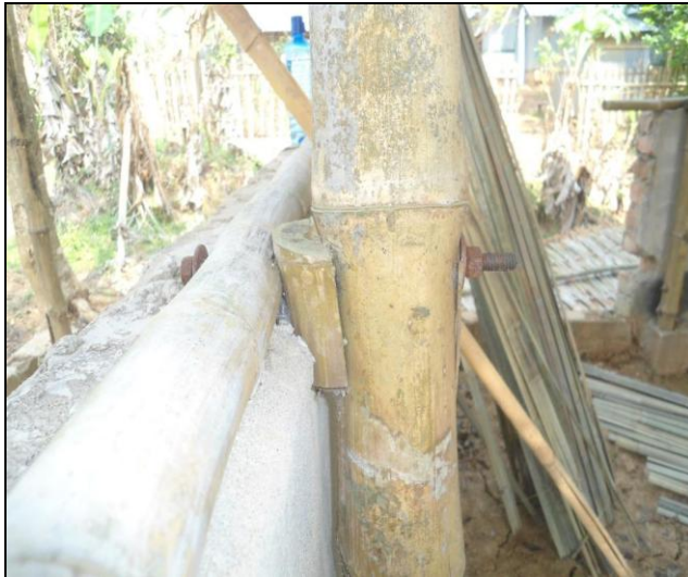
A section of bamboo can be used in case a bolt length go excess
