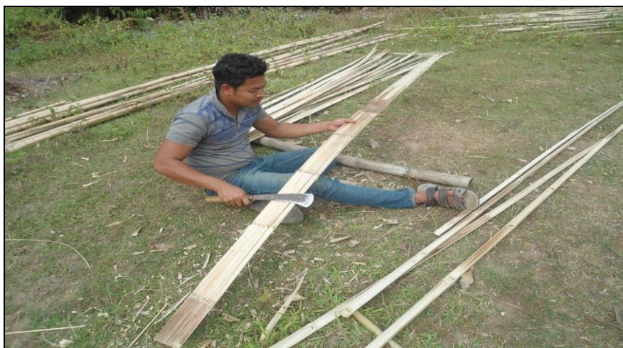
Making the bamboo splittings/torja for house wall construction
