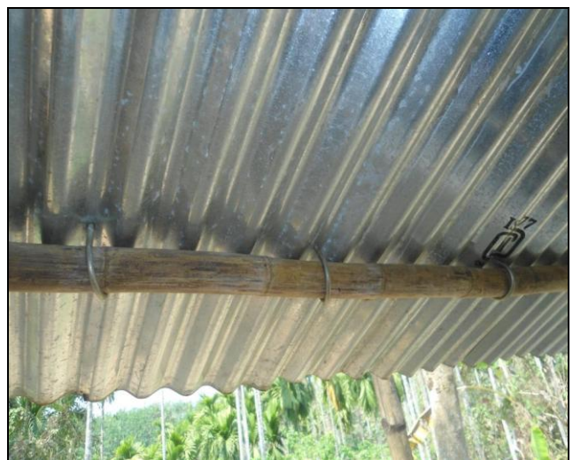
3: Putting metal cap, bitumen washer on the J-Hook and fastening it with nut
