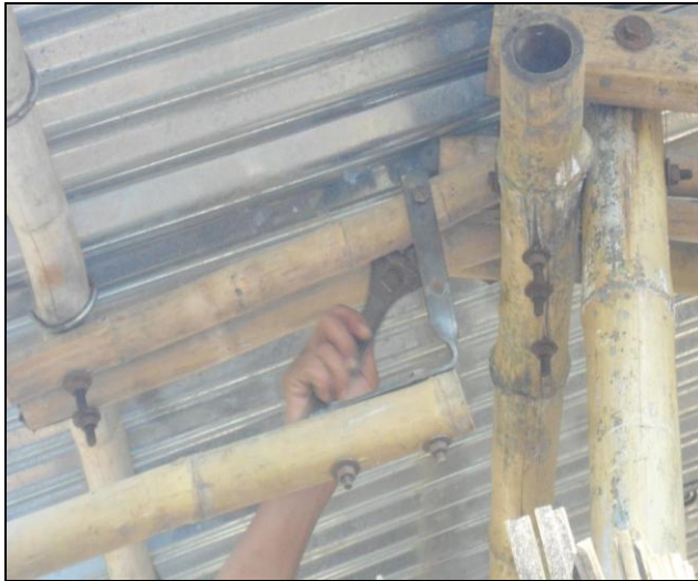
7: Joining of the clamp fixed on Kanakaich bar with the truss on the main building
