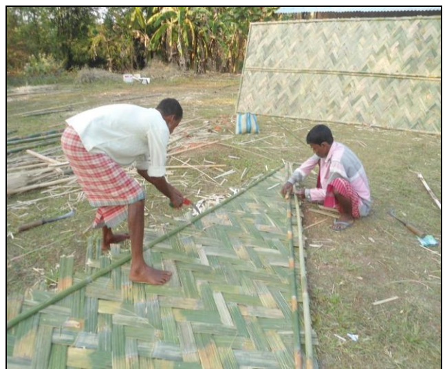
Tightening the wall structure by GI wire
