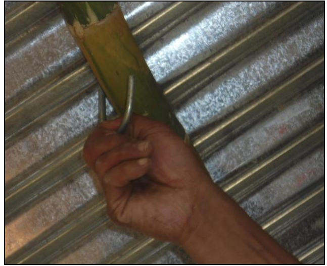
2: Inserting the J-hook from below
