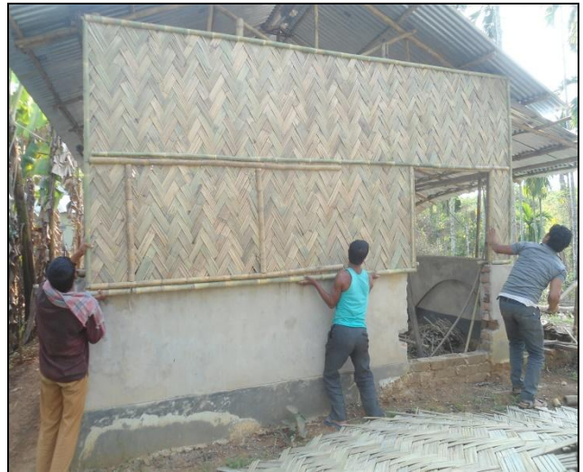
Fitting of bamboo wall on the house
