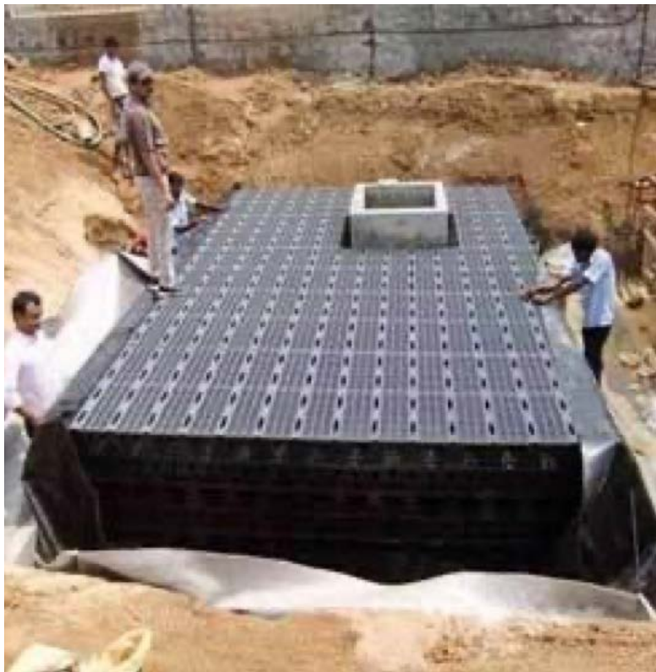
Figure 66: Groundwater Reservoir,, Sekisui Cross Wave Rainwater Harvesting System ( https://www.indiamart.com/proddetail/sekisui-cross-wave-rainwater-harvesting-system-3693210291.html )
