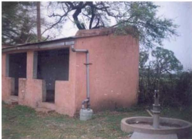
Roof top rain water harvesting in villages of Madhya Pradesh
