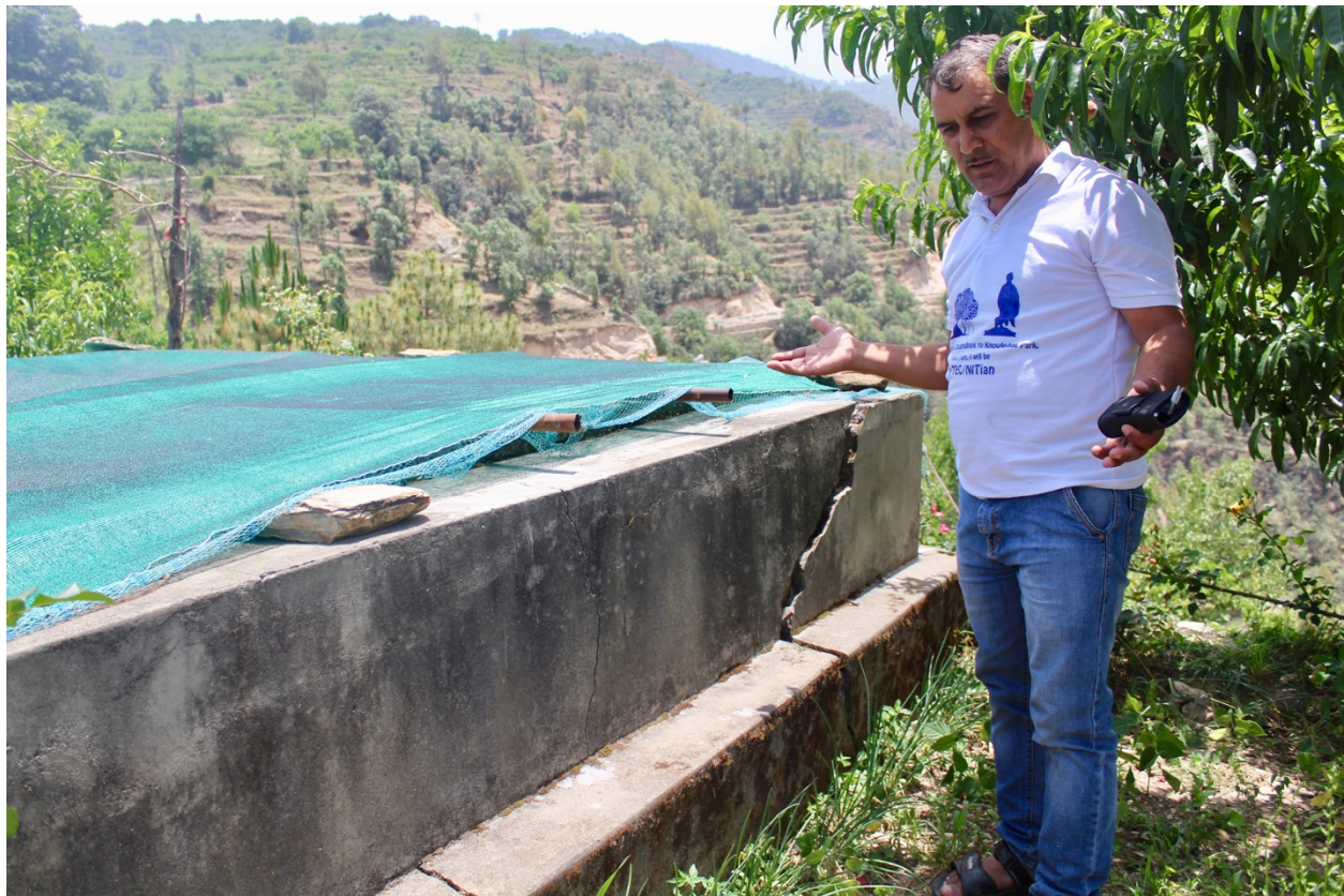
Figure 5. A cracked concrete tank that has been repurposed and lined with polythene as part of the project.
